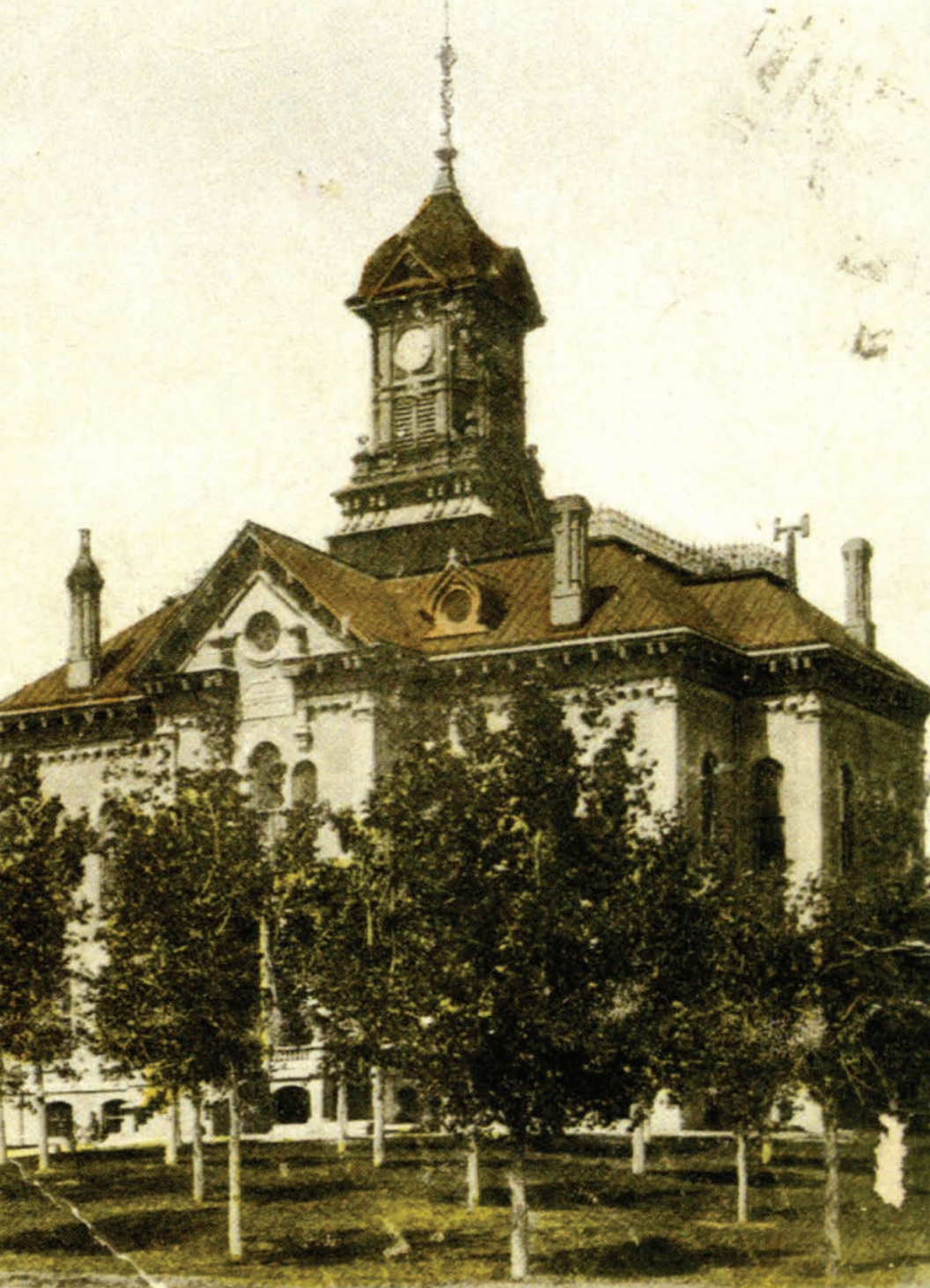
HUGHES COUNTY COURT HOUSE, PIERRE, S. D.
